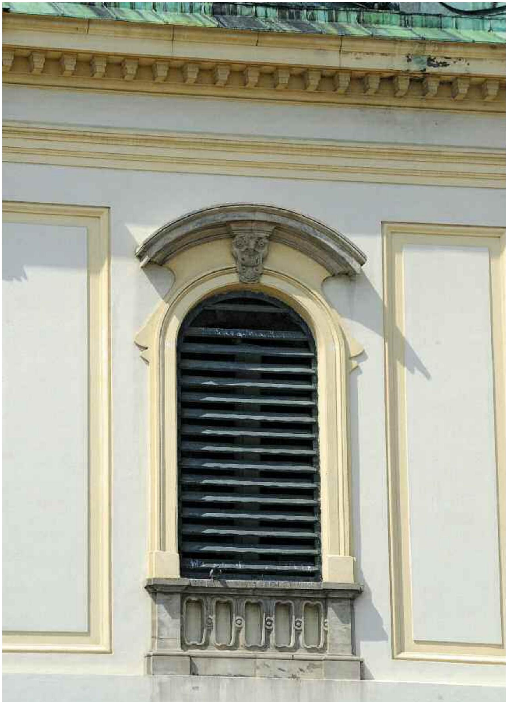
10, 11 Framing of the bell opening; Corinthian capital and entablature on the third storey of the southern tower, before 1737, designed by Giuseppe Fontana II
