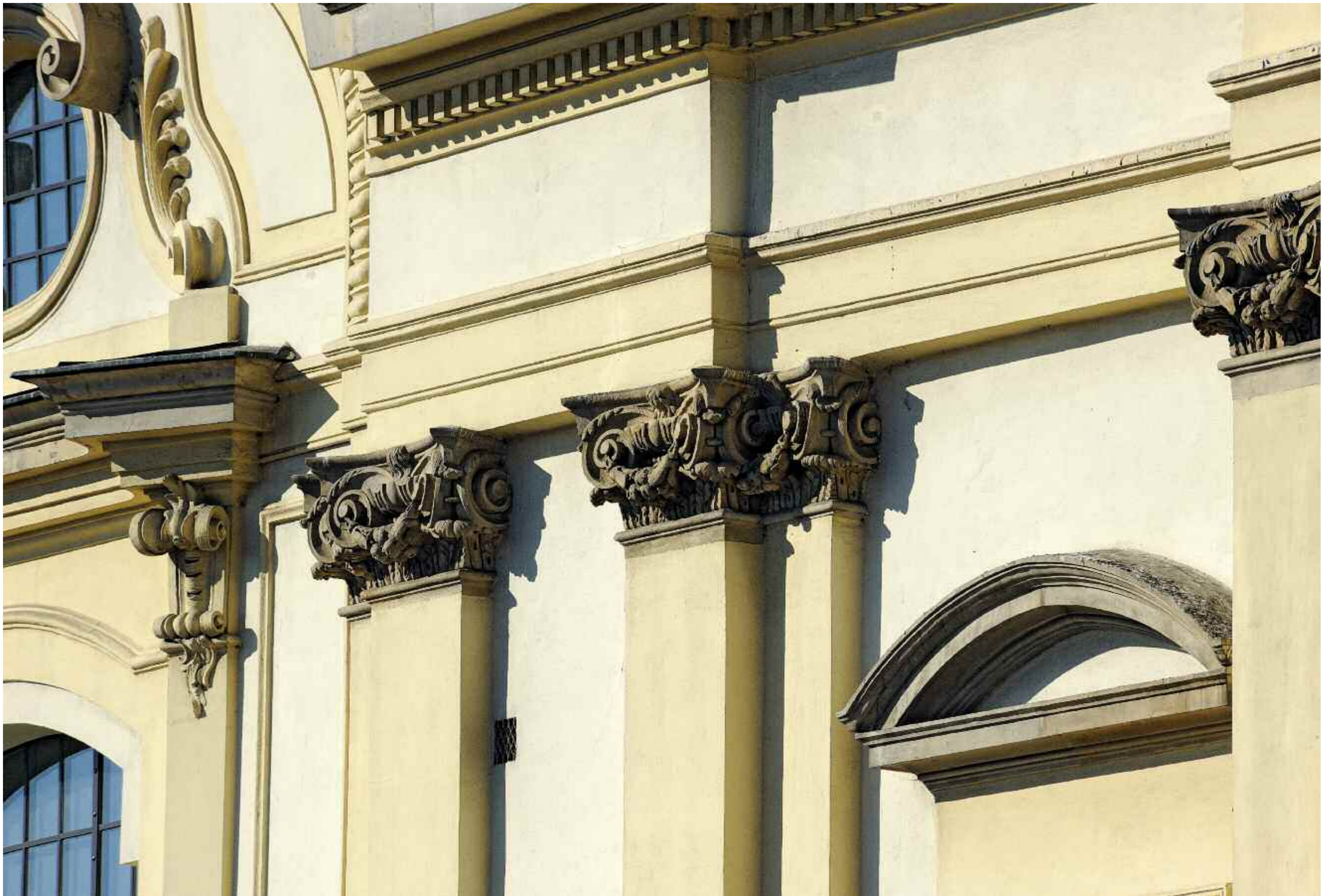
9 Perspective view of the articulation divisions of the second storey of the façade
