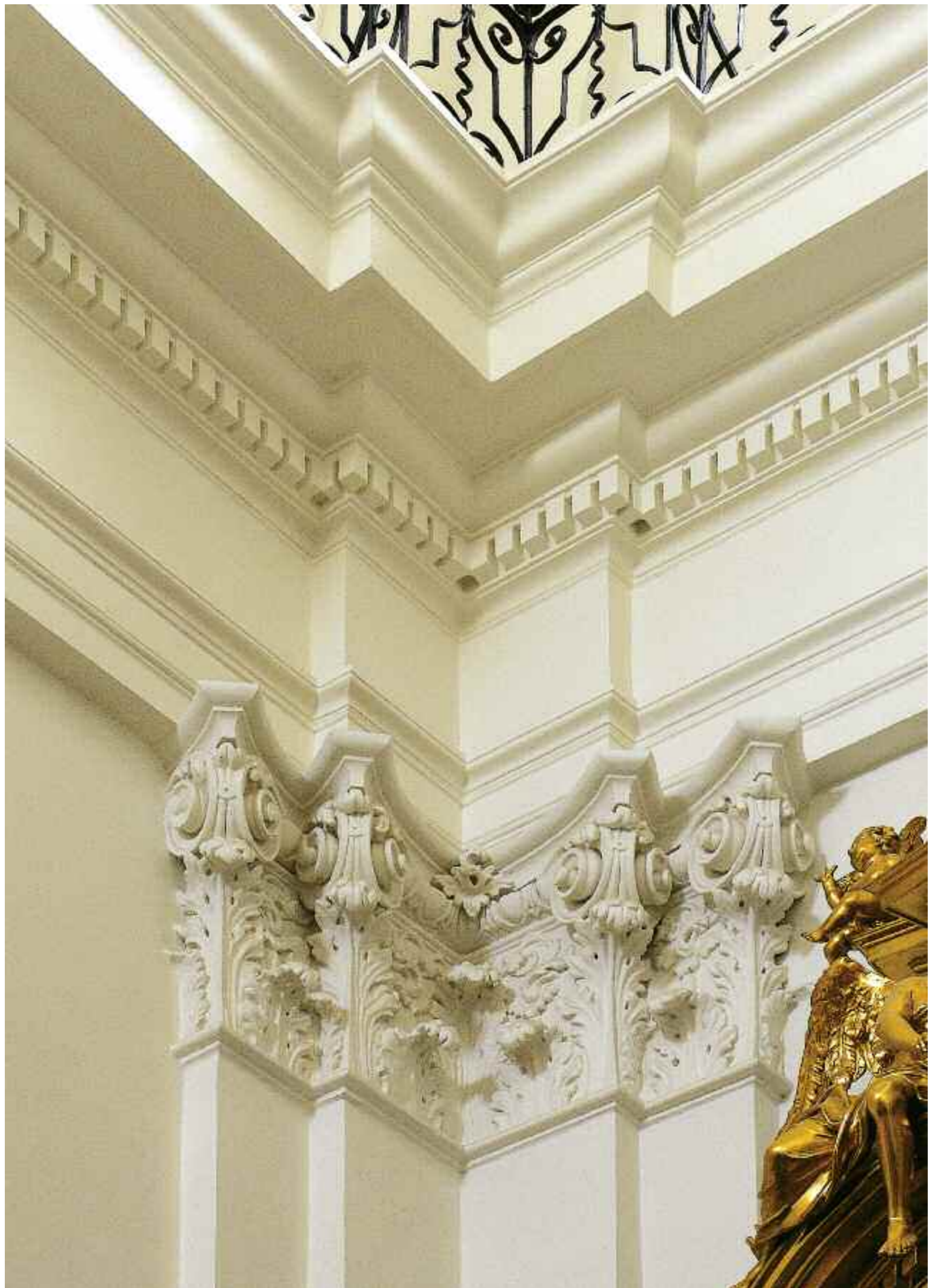
63 Stuccoed Corinthian capital in the corner of the Chapel of St. Charles Borromeo (St. Joseph), 1690s, designed by Giuseppe Simone Bellotti
