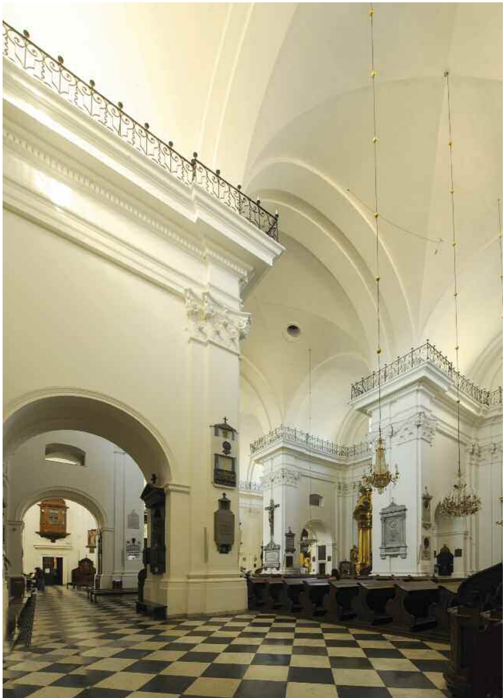
20 Panoramic view of the partitioning wall-pillar structure of the Holy Cross interior from the Chapel of the Archangel Michael
