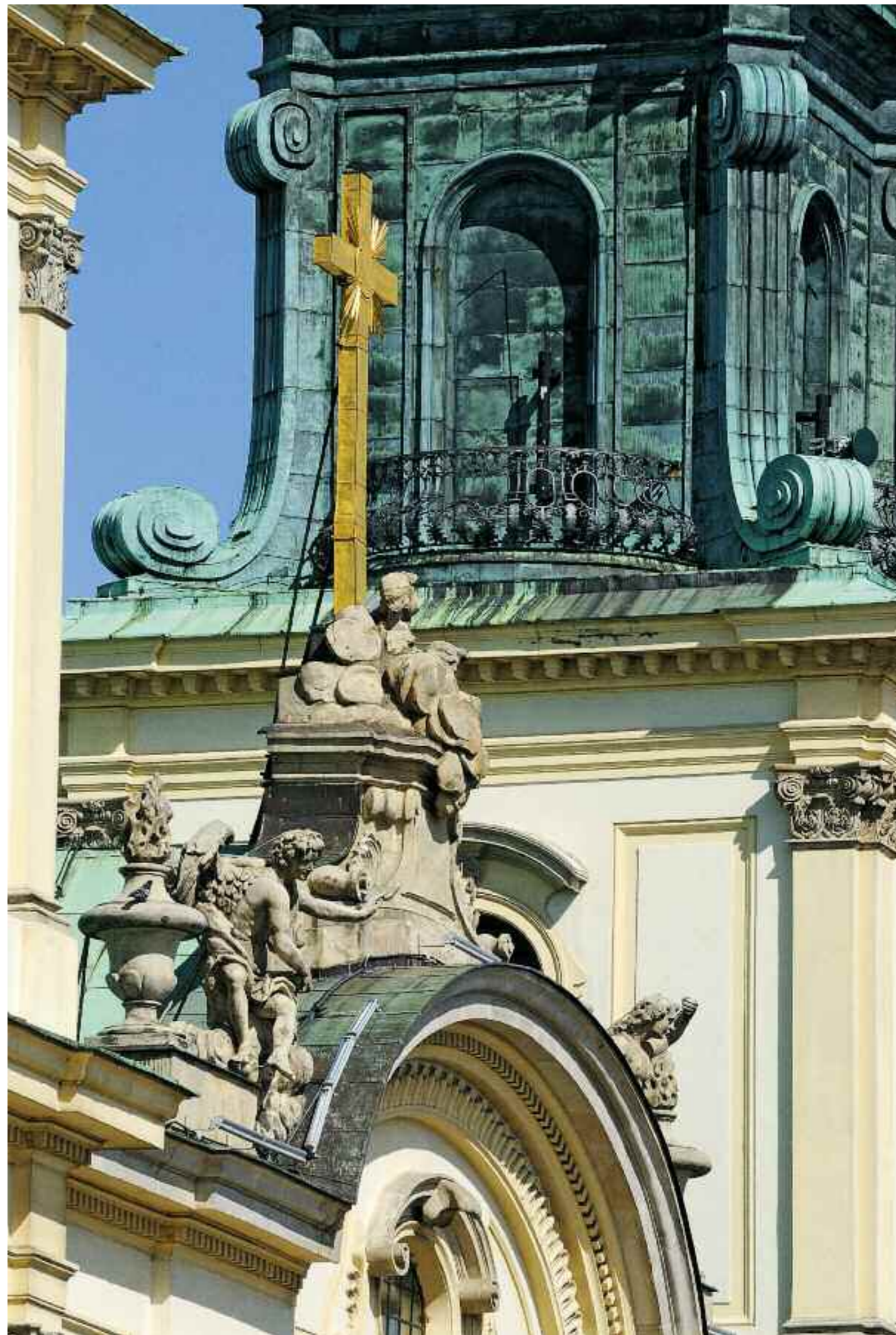
8 Perspective view of the facade finial and the northern tower
